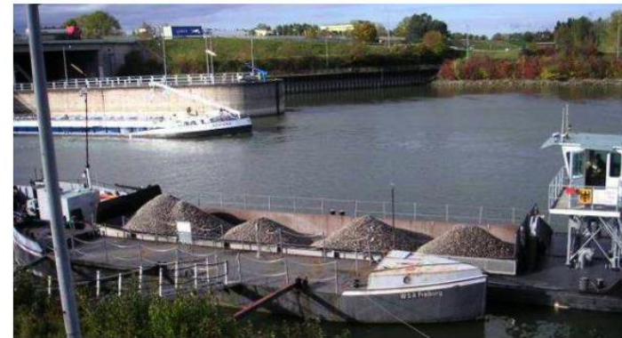
Figure 10. Nourishment of the Rhine River by barges of gravel.
