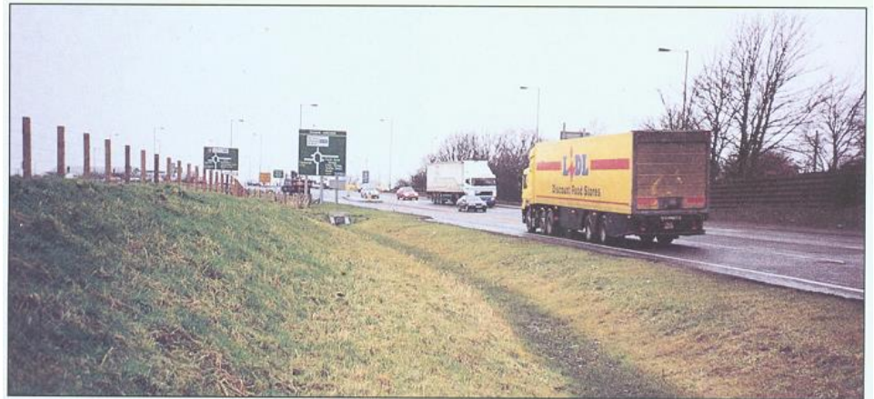
Swale on A8000 near Edinburgh. No kerbs or gullies are required.
